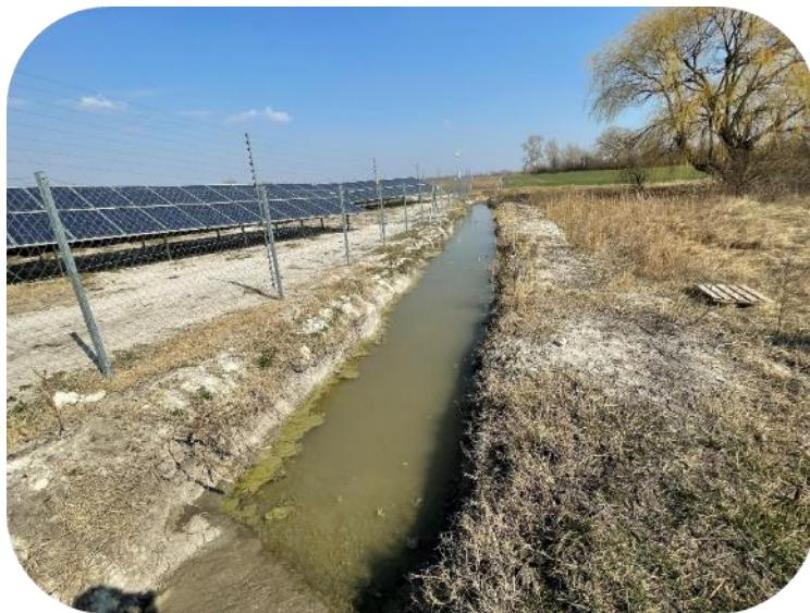
**Fig. 2. The current precipitation collection ditch created in sample area No. 2.**
